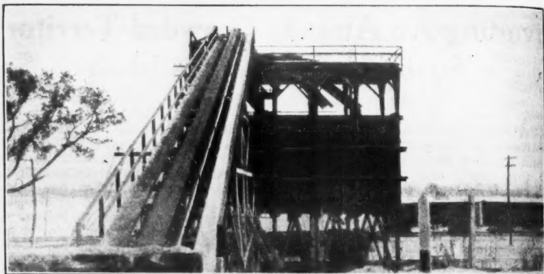
Bunkers Viewed from State Highway
